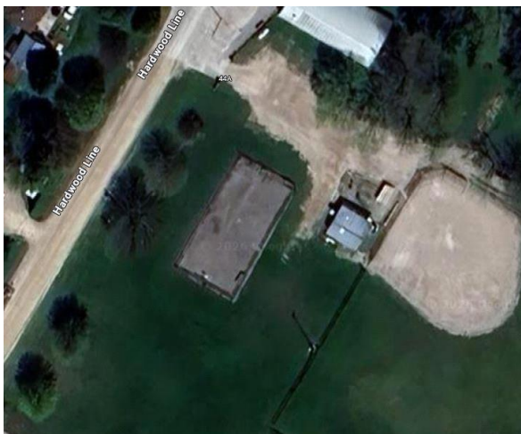
Aerial picture of Auburn Sports Pad.
