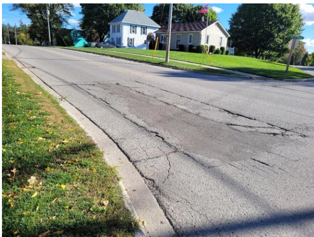
Large alligator cracking and potholes.
