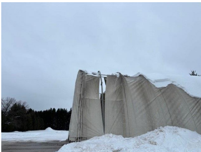
Image of torn tarp on Londesborough Road Shed coverall.
