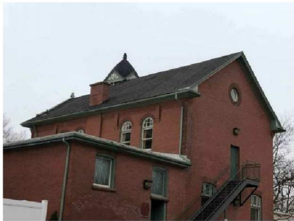
View of South East Corner
