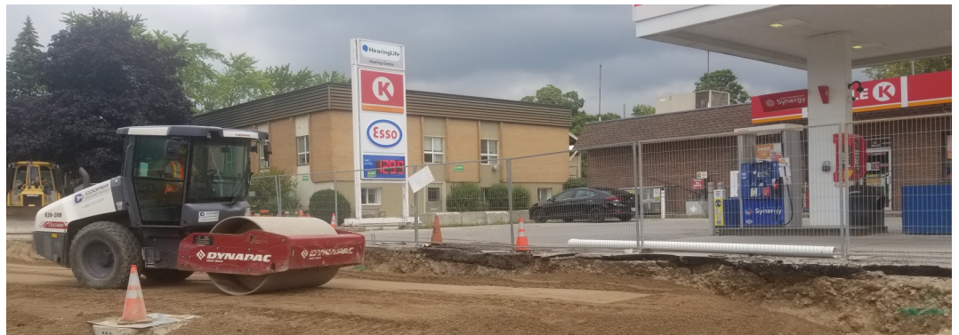
New temporary access driveway being built for Esso
