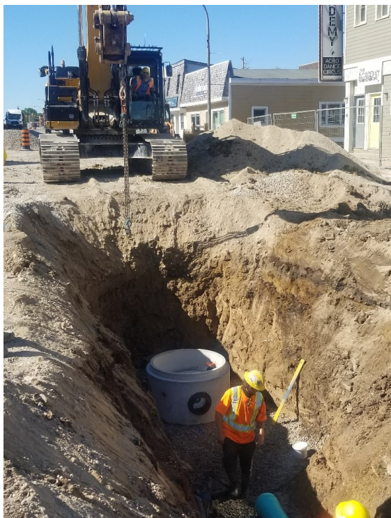
A manhole being installed, with a new sanitary sewer pipe waiting at his feet.
